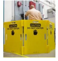
An unqualified worker may not understand the boundary system; therefore, use additional means to impede the unqualified worker from entering either the Limited Approach Boundary or the Arc Flash Boundary. The primary means of preventing access shall be a barricade system. Barricades should be
